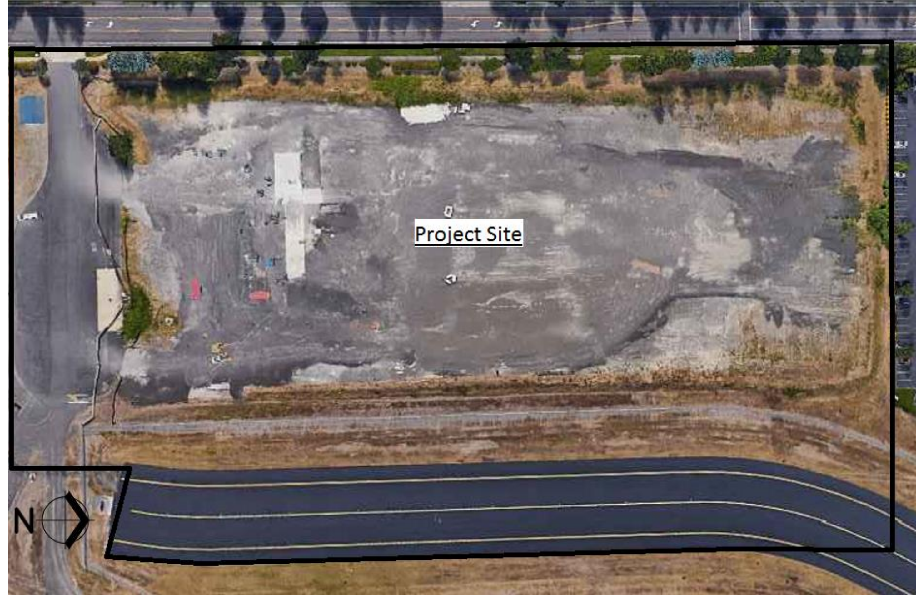
Figure 3. Aerial of Project Site and Taxiway J
