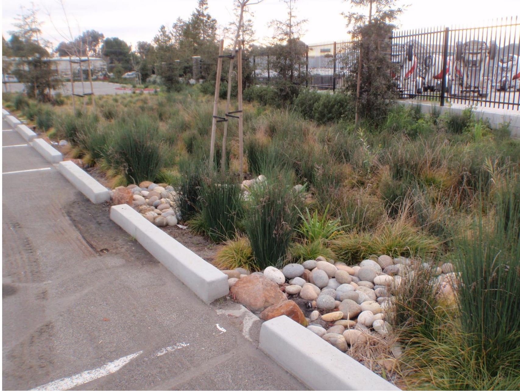
Figure 1. Example of a Rain Garden Stormwater Treatment System
